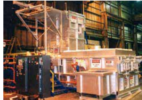
Figure 8 — Schematic of Jet Melter™ above and an actual example of one installed below.
